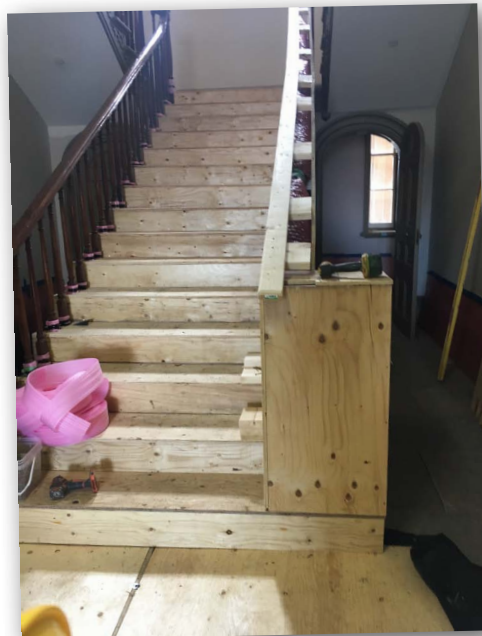
Main staircase from the ground floor
