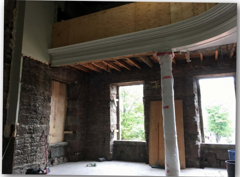
The Chamber with finishes removed to expose interior walls and structures
